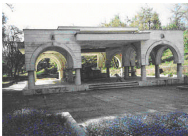
Figure 13 Thermal water fountain (Hisarja town).
