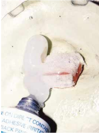
Fig. 6. Silicone applied to resin substructure and polyurethane lining.
